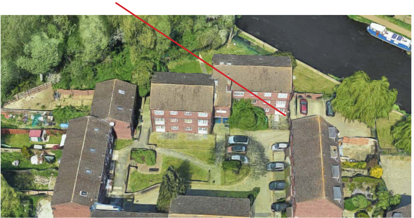
Image 3. Aerial view of current site
